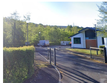
Augusta House, Ebbw Vale
